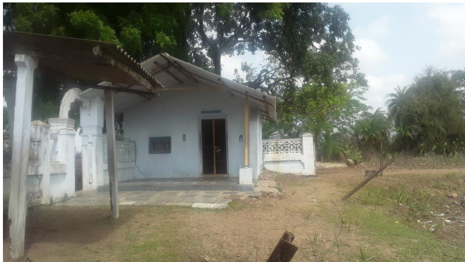
Pictures of Kavutaram First Railway Station –‘Kavutaram Gate’
